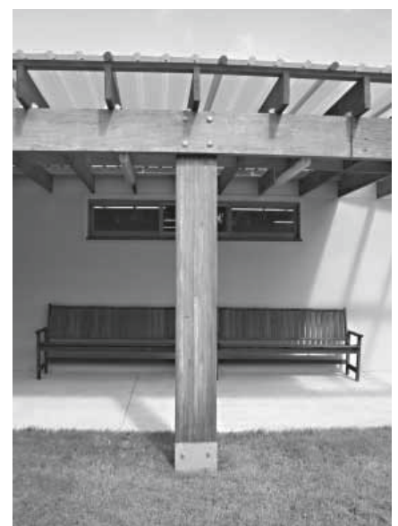
From top: Water tanks capture rainfall from the large roof area; visitors reception; solid timber posts and pergola outdoors.
